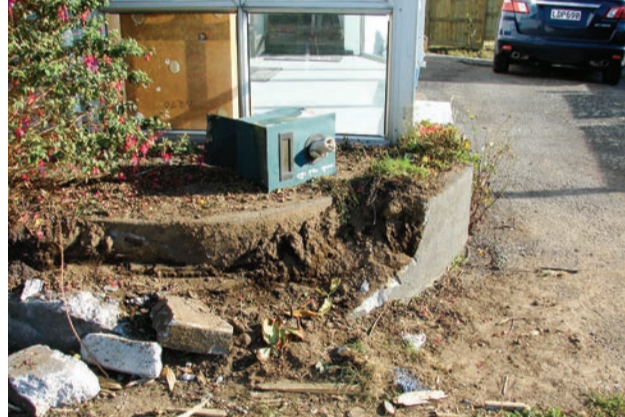
The truck clipped the concrete garden boundary, just missing the house.
